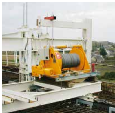
Brokonstruktion. Bridge construction.
