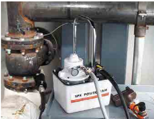
▶ The PA17 used with a flange spreader
